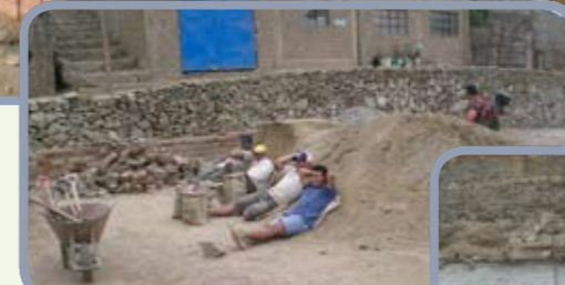
Photos: Building the newest addition to the medical centre.
